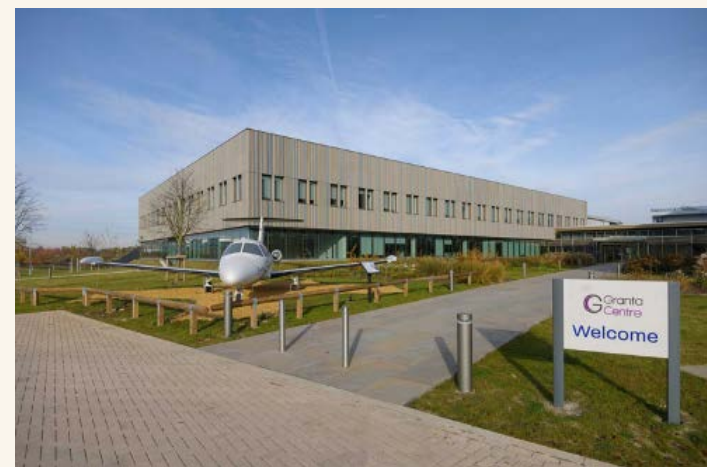
Granta Centre, Granta Park, Granta
