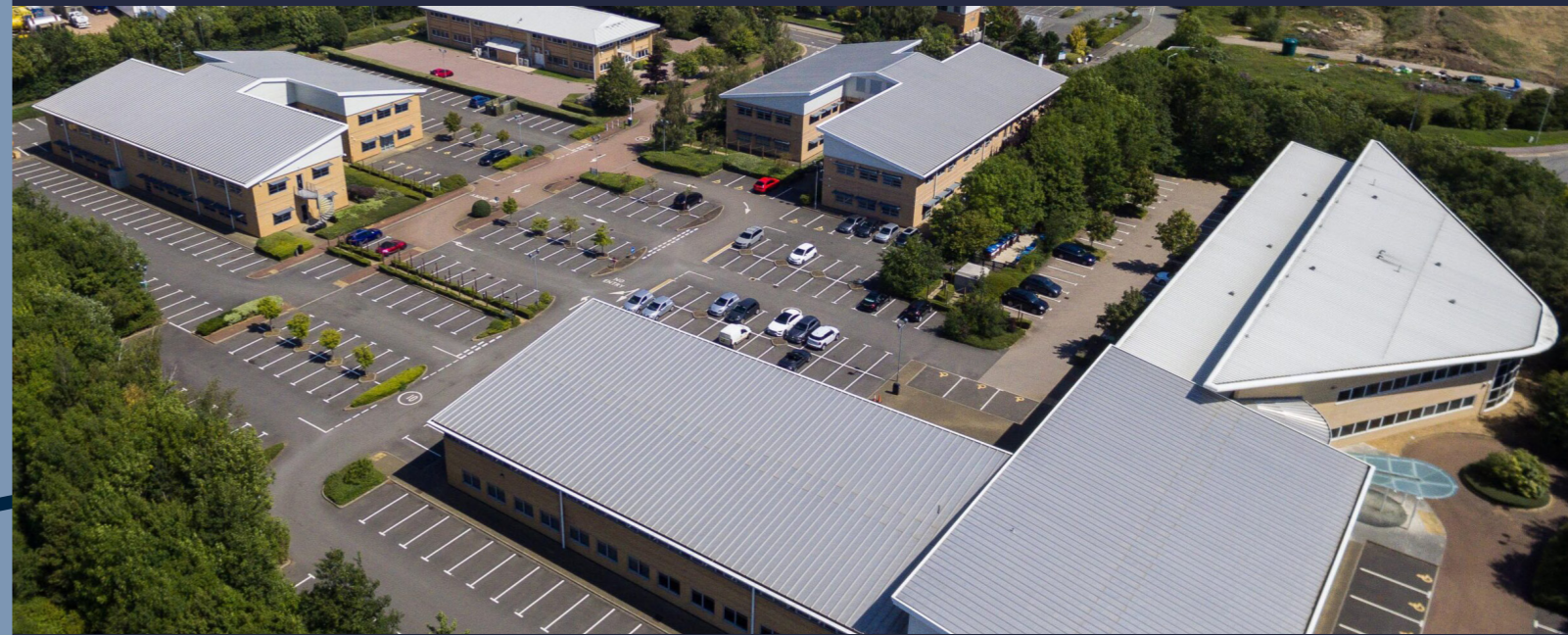
Aerial view of Cranfield University Technology Park
